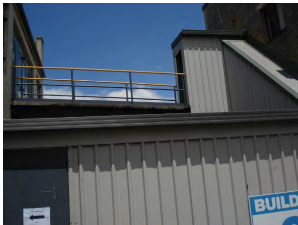
Bridge connecting Building 1 & Building 2A, L2.
