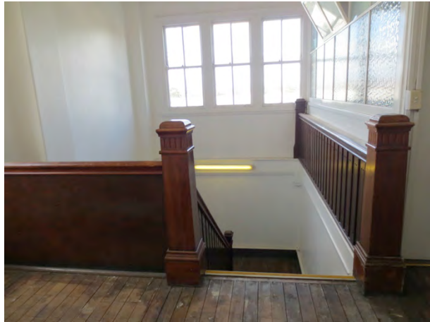
Building 2, L1, timber stair.
