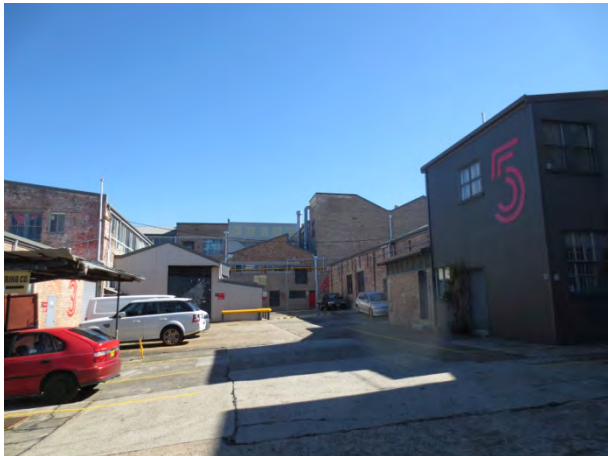
Building 5 south elevation, looking west.
