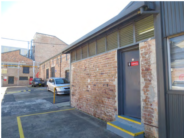
Building 5B, south elevation, looking west.
