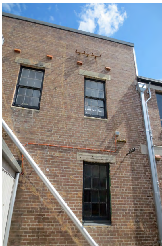
Building 1D, showing ceramic insulators that should be retained.
