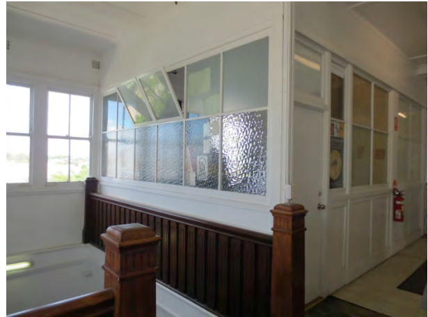
Building 2, L1, timber stair + office room. These elements should be retained if possible.
