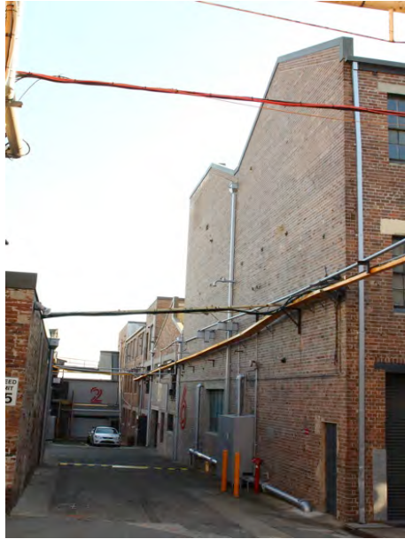
Building 6B east elevation, looking south.
