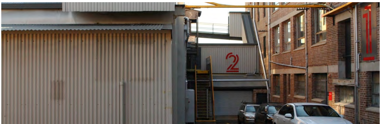
North elevation Building 2A in the distance.
