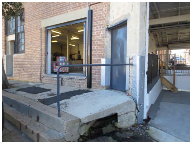
Loading bay on Mary Street, Building 1D with Building 2A in background.
