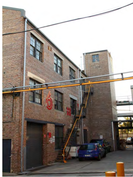
Building 6B north elevation, looking west.
