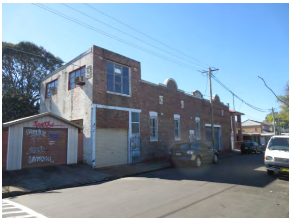
View north on Edith Street showing 1918 warehouse building opposite the site.
