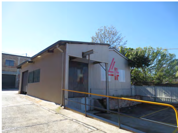
Building 4 looking north.
