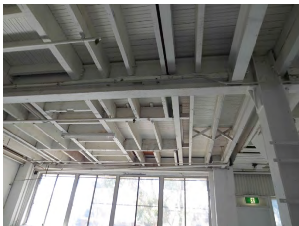
Building 7, G, Tenancy B7 F2, showing ceiling.
