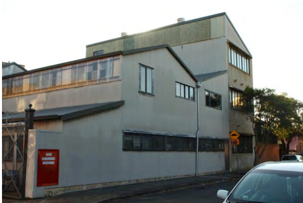
Building 7C & 7B north elevation.
