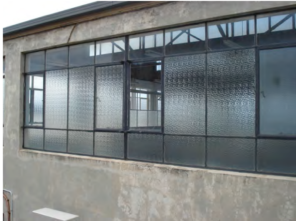
Building 2A, north elevation window detail L2.
