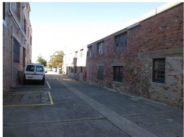
Between Building 5A and 8, looking east.
