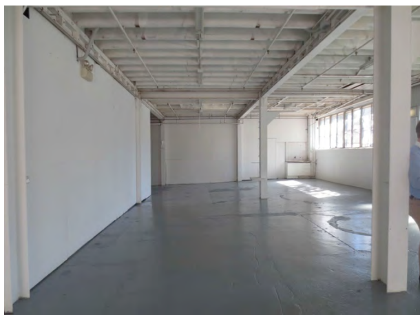
Building 7, G, Tenancy B7 F2, looking west.
