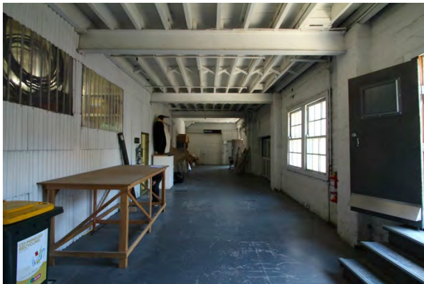
Building 6, LI, Common Area, looking west.
