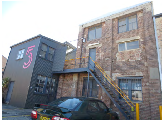
Building 5D & 5C south elevation, showing external stair.
