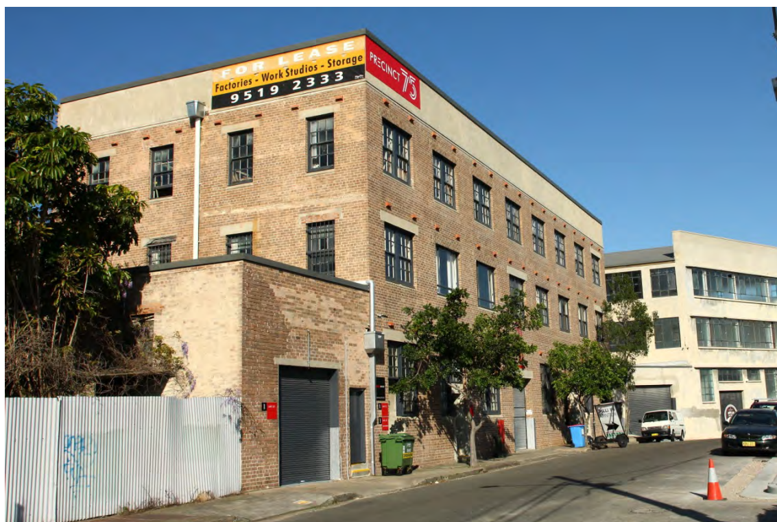
View looking east along Mary Street, Building 1C in foreground, Building 1D in middle and Building 2 in background.
