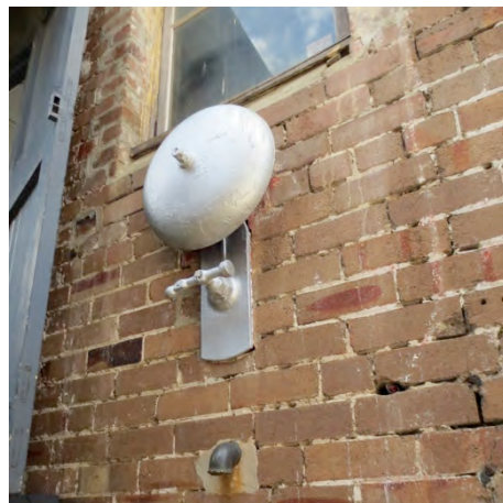
Building 3B, large fire bell that should be salvaged and relocated.
