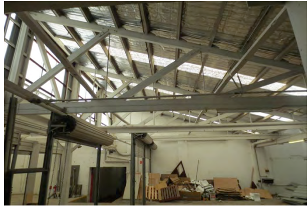
Building I, Ground level showing timber trusses + steel rod construction.
