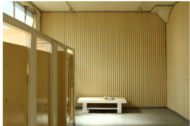
Building 8, L2, Shared Toilets, looking south.
