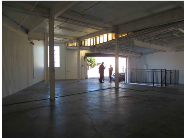
Building 2, G, Tenancy B2F1, currently unoccupied looking south towards Mary Street.
