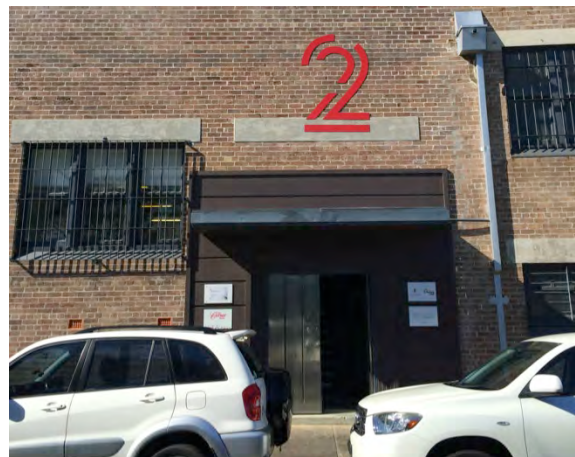
Detail of entry, Building 2A.
