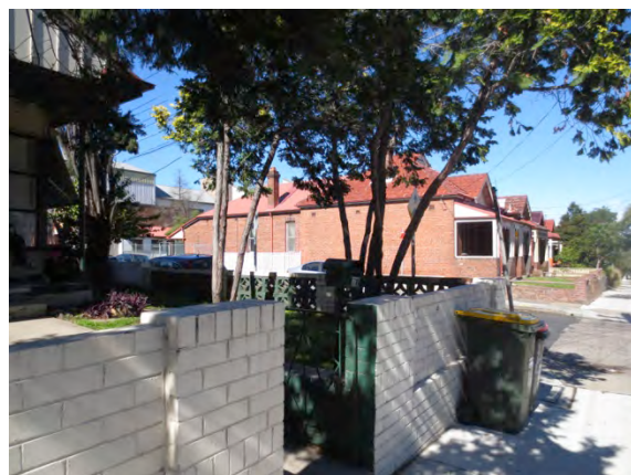
View south on Unwins Bridge Road showing single storey brick terrace housing.
