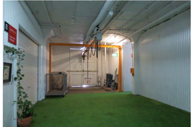
Building 8, L1, Common Corridor, looking south.
