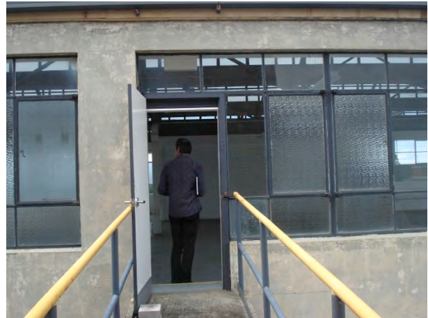
Bridge connecting Building 1D & Building 2A, L2.
