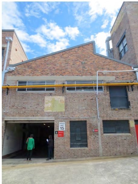
Building 6C. This section of the building is a later addition.
