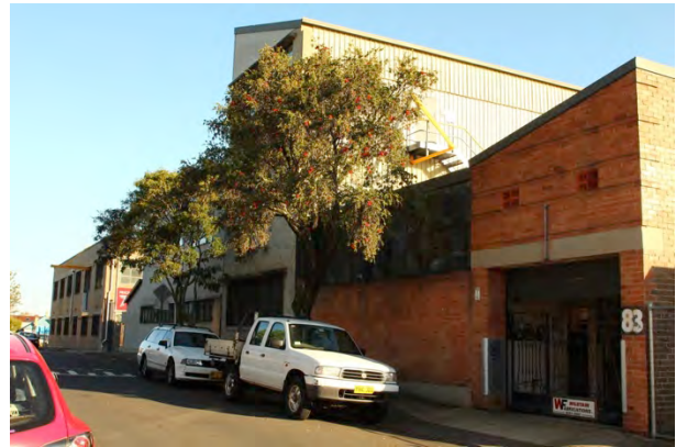
Building 7C, 7B & 7A north elevation.
