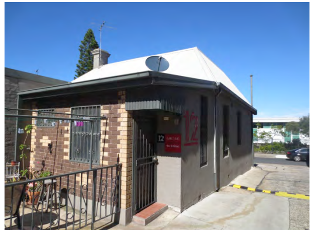
Building 12, North & West elevations.
